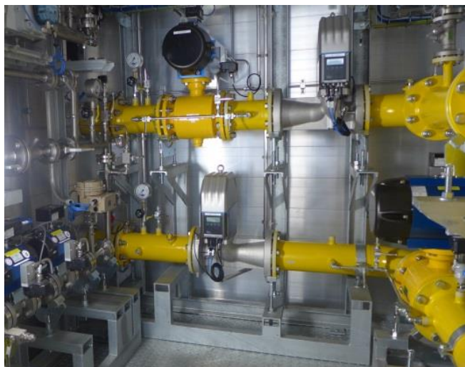
Feed-in plant mixing hydrogen into the gas mix while maintaining the characteristic/threshold values of the natural gas grid. ©Fraunhofer ISE
