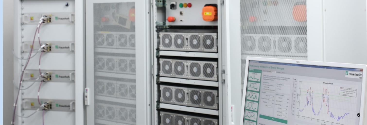
systems. The converters were deployed to interconnect a battery storage unit and a wood-working tool machine. Besides providing resiliency, the deployment of the active controlled storage system contributed to improve the total energy efficiency of the machine by up to 10 % by regenerative braking energy that would otherwise be dissipated into heat.
