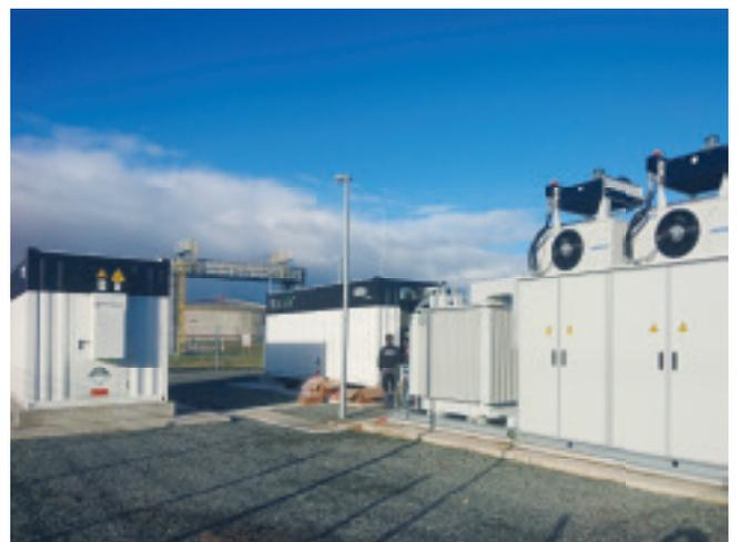
*Figure 4: Battery electrical storage system for frequency stabilization*
