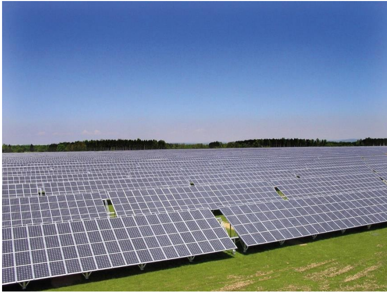
Photovoltaics is the main pillar of the energy transition. ©Fraunhofer ISE
