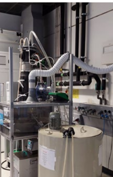
Methanogenic stage of anaerobic biogas installation with fixed-bed circulation reactor.
