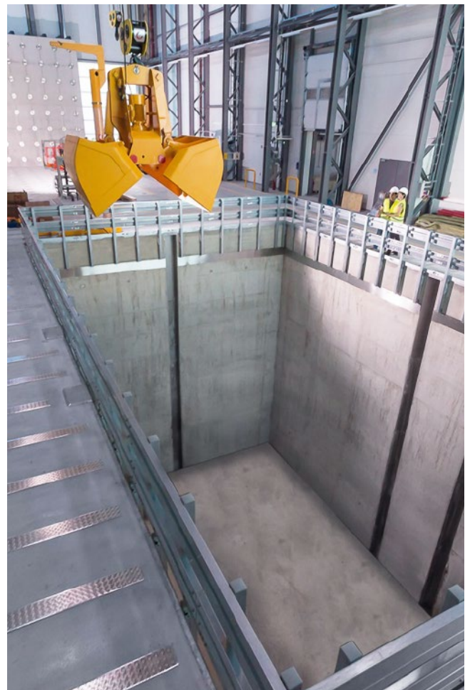
THE TEST PIT FOR OFFSHORE SUPPORT STRUCTURES HAS A VOLUME OF 1,260,000 LITERS. That is the equivalent of around 90 truckloads of sand.
